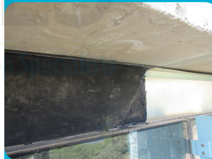
Glazing Head Details- Designed for Large Tolerances
